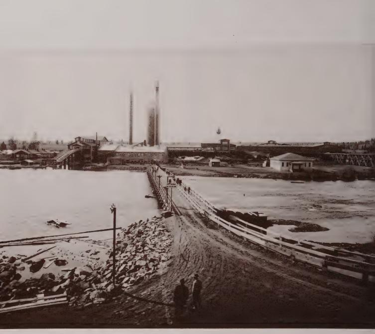
The Shevlin-Hixon's million-dollar burner was over 100 feet high, was built with fire brick four feet thick, and was covered with one-half and three-fourth inch steel plates. When the mill closed, the burner was scientifically dynamited, and the steel was sold to sheep ranches to be used for water tanks.
