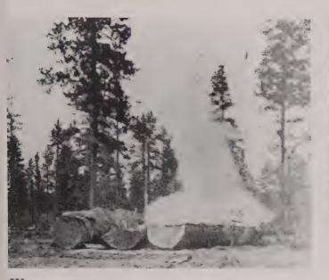
With only one charge going off the log was split neatly in half with very little lumber wasted and two halves much easier to load on flat cars.
