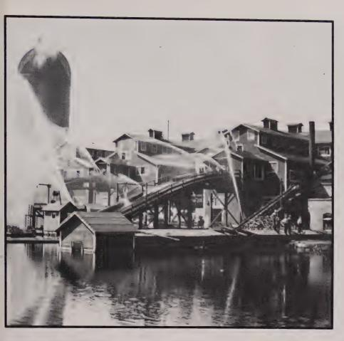
Shevlin-Hixon is shown with the mills cutting. Streams of water wash logs going up the chutes, because dirt and debris dull the saws. From the author's collection
